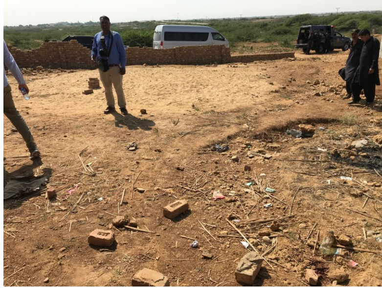
The multi-purpose hall is to be built on the light sandy area behind the photographer.
