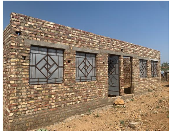
New classrooms, still unfinished
